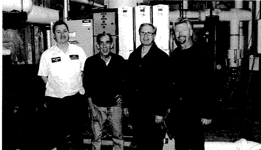
(R to L) Chief Engineer Tom Wojciechowski, Plumbing Contractor Bob DeGuiseppe of Chicago-based Great Lakes Plumbing, Architect John Kowalski of Klein and Hoffman located in Chicago and Plumbing Engineer Kent Locke, Jr., of Fox Valley Engineering in Fox River Grove, IL.
